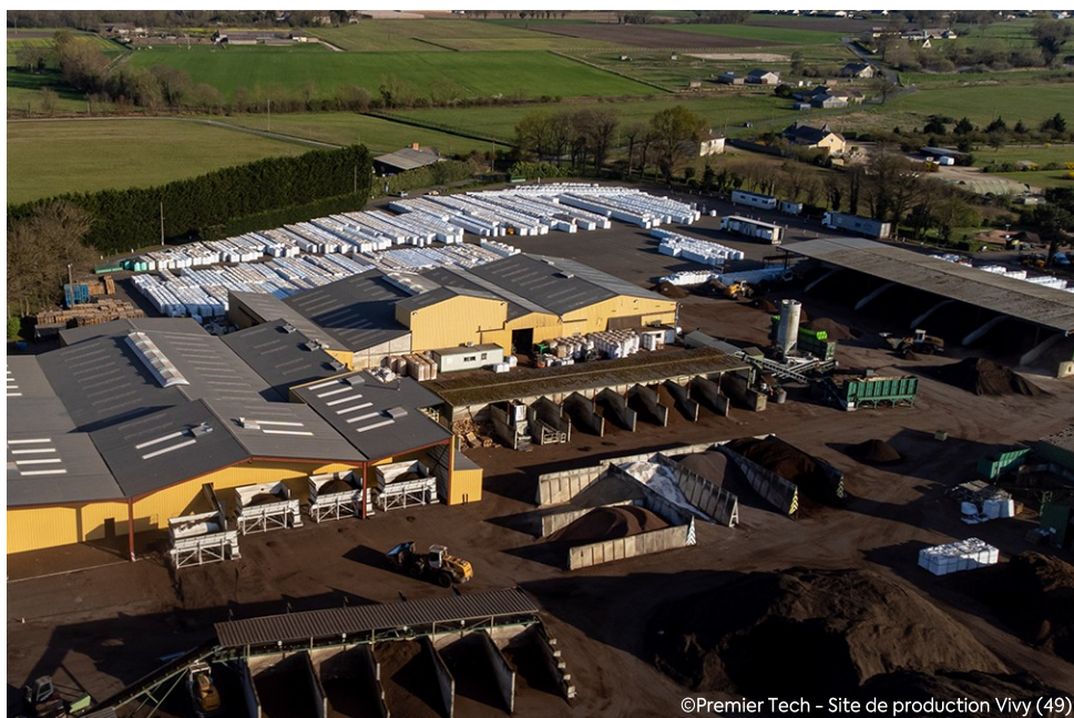
©Premier Tech - Site de production Vivy (49)
