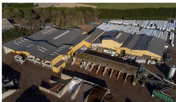
©Premier Tech - Site de production Vivy (49)
